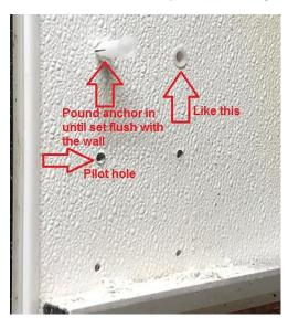
6. Attach Wall Mount (H) to the wall using 6 anchors (F) and 6 lag screws (I). The lag screws can be driven into the wall using the drill and 10mm socket or Phillips head.
